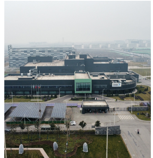
Our LEED Gold-certified Xi'an, China, Janssen facility with a 1 MW solar array installed in 2020.
