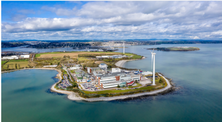
Wind turbines at Johnson & Johnson's facility in Cork, Ireland.
